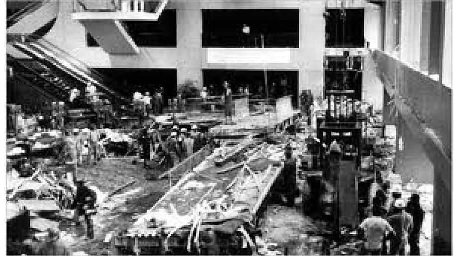
Three days after the disaster a structural engineer discovered a significant change of the original design of the walkways. This design change would prove fatal.
